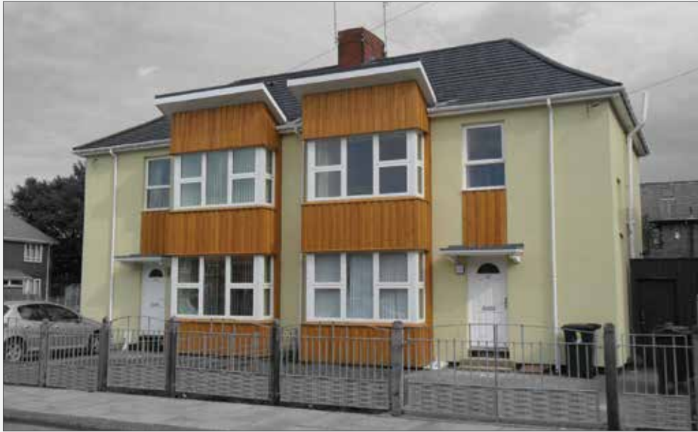
Figure 12: Bay window module and roof pod
